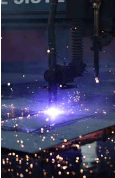
STEEL PRE-FABRICATION WORKSHOP
